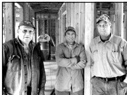
From left, John Kuebrick, Donnie Niehoff, and Steve Batusic pausing from getting the walls up in November, 2013.
